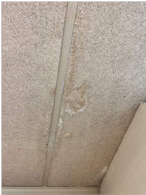
Photograph 3. Water staining on fibrous ceiling
